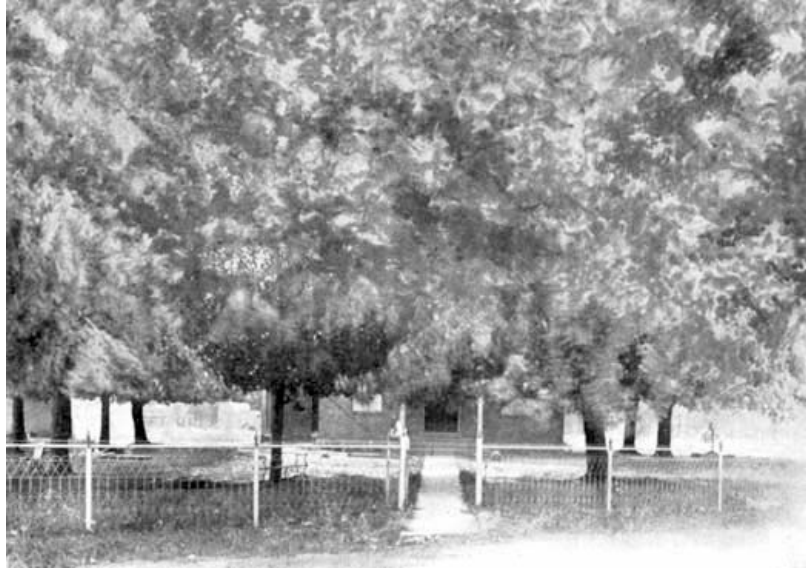
A COUNTRY SCHOOL BUILDING.
