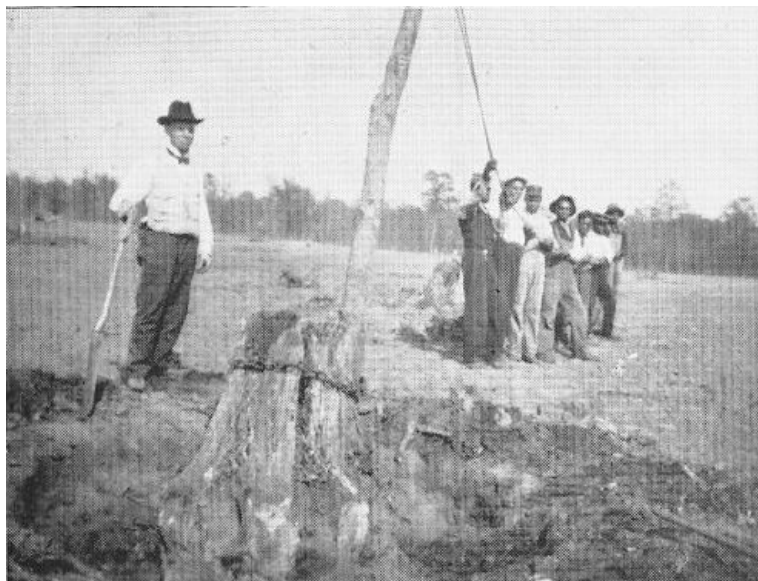
READY FOR A PULL
