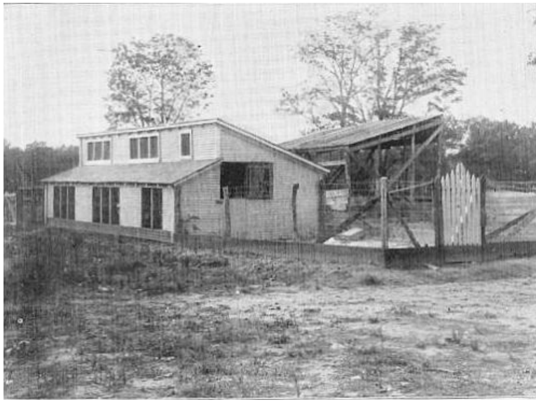
THE HEN HOUSE; OPEN FRONT, SEMI-MONITOR ROOF
