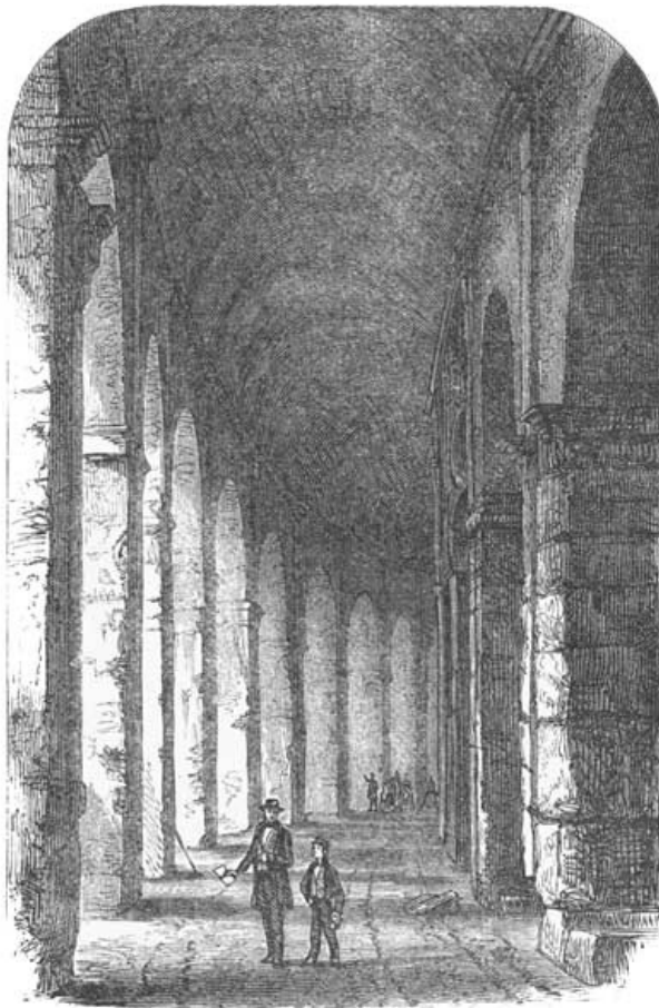
VIEW OF THE LOWER CORRIDOR.
