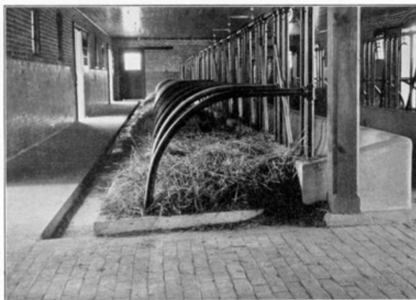
CONCRETE STABLE FLOORS.
