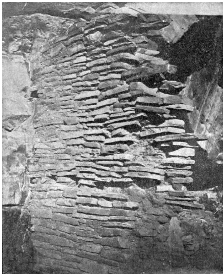
Fig. 250—Structure of wall of Honanki
