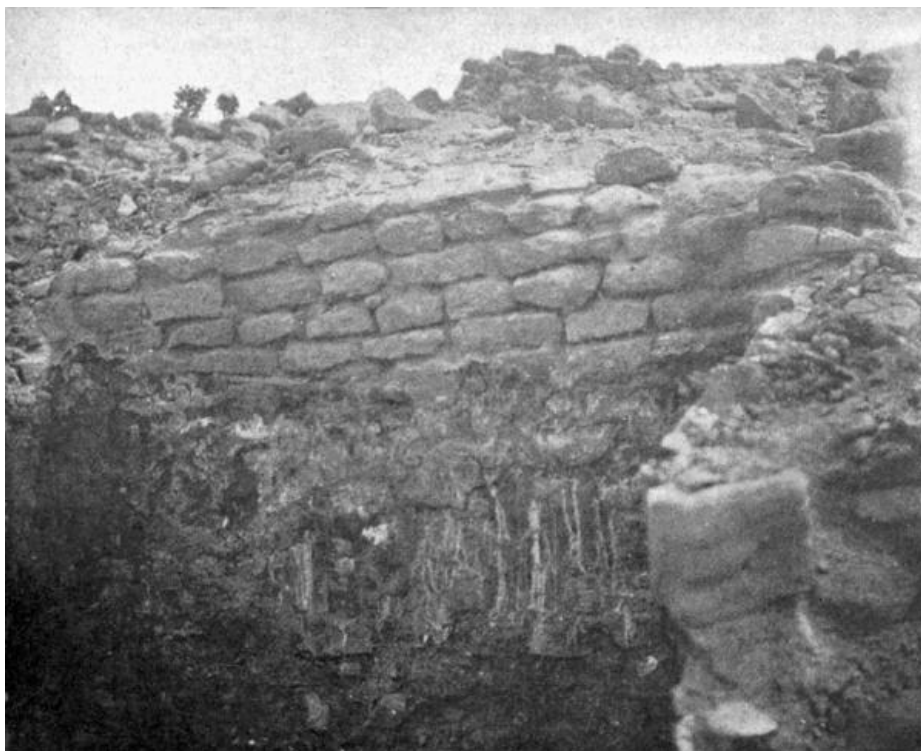
Fig. 256—Structure of house wall of Awatobi
