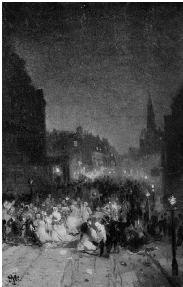
STREET SCENE DURING THE CHARLESTON EARTHQUAKE.
