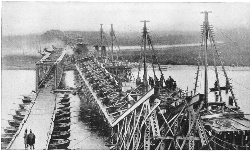
A bridge on the Kalesch-Warsaw line blown up by the Russians in their retreat toward Warsaw. At the left is the pontoon bridge built by the Germans
