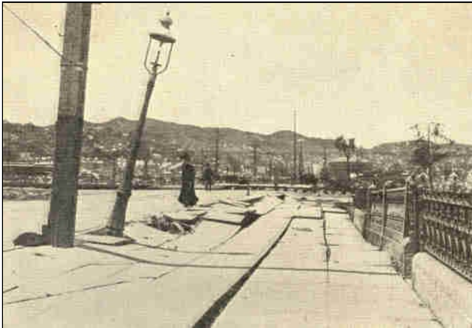
Earthquake at San Francisco, April 18, 1906.
