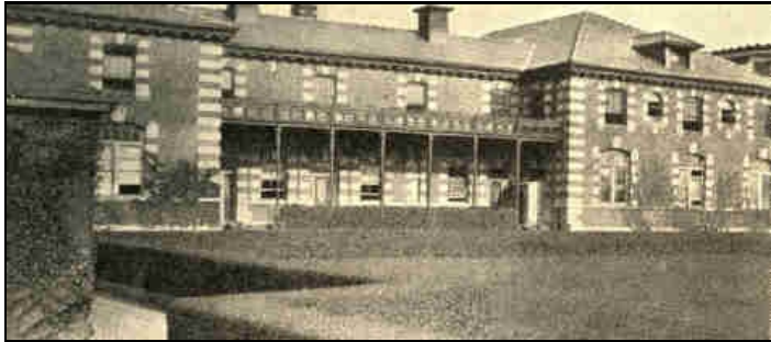
Restaurant. Immigrants dining-room and detention quarters.
