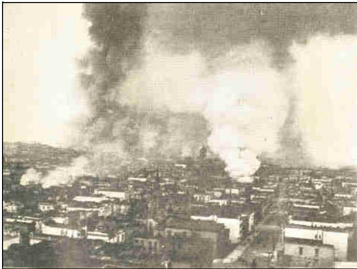
Showing destruction of buildings after the earthquake and fire in San Francisco.
