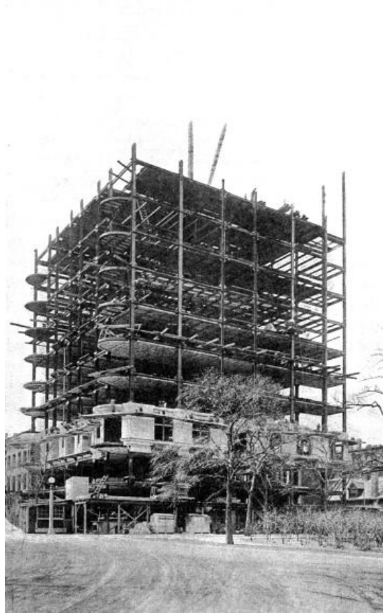
A STRUCTURAL STEEL APARTMENT BUILDING
