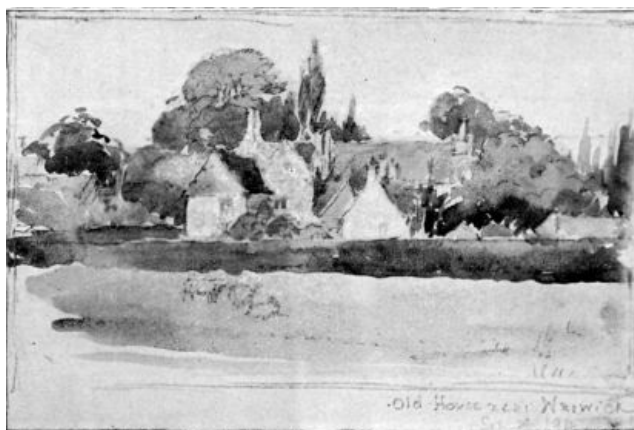
OLD HOUSE NEAR WARWICK. SKETCH BY WILSON EYRE, Jr. From The Architectural Review , Vol. IV, No. 1.
