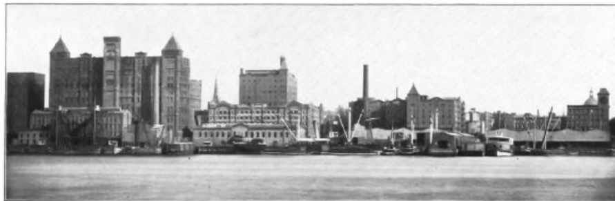
HAVEMEYER SUGAR-REFINERY, BROOKLYN, N.Y.
