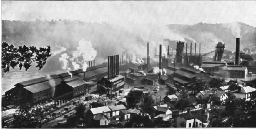
STEEL MANUFACTURE—THE NATIONAL STEEL COMPANY'S SMELTERY AND ROLLING-MILLS, MINGO JUNCTION, OHIO
