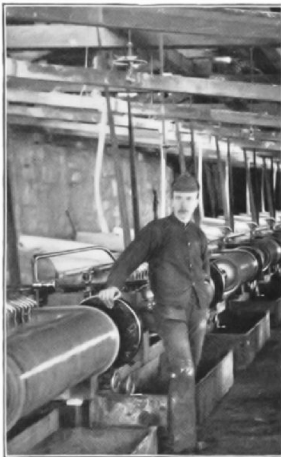
INTERIOR OF MILL
