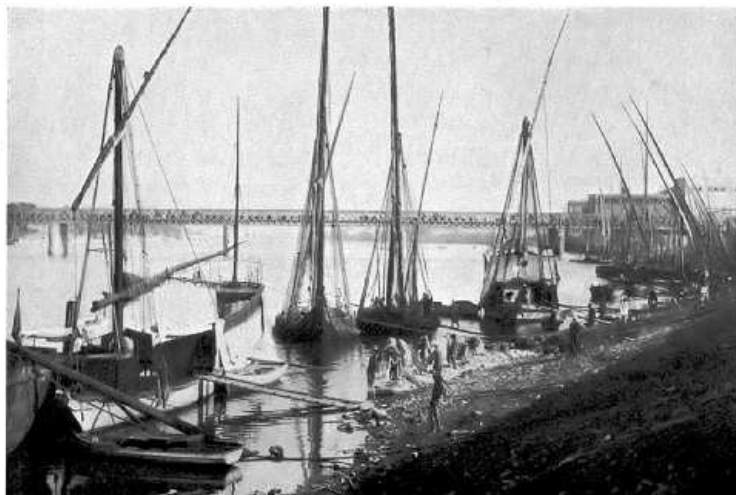
A bridge spanning the Nile at Cairo
