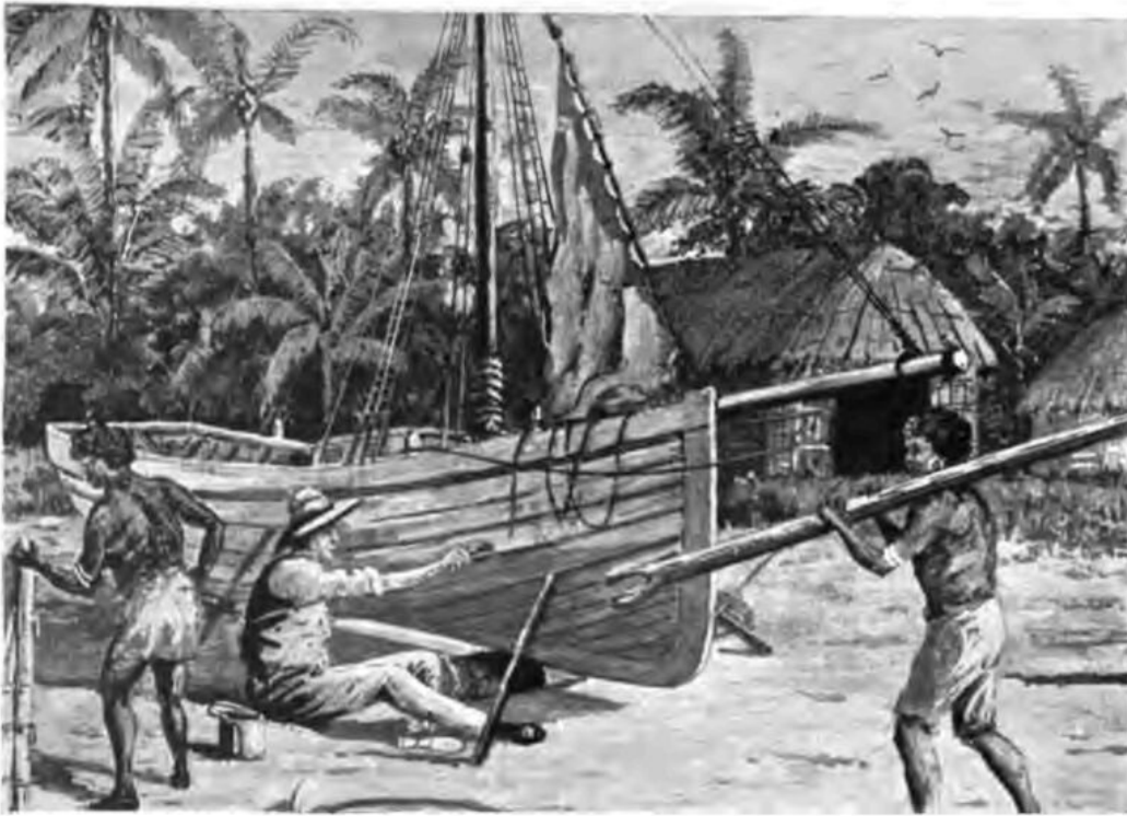
THEN I GAVE HER TWO GOOD COATINGS OF RED LEAD FROM KEEL TO ABOVE WATER LINE, AND, ABOVE THAT, PAINTED HER WHITE.
