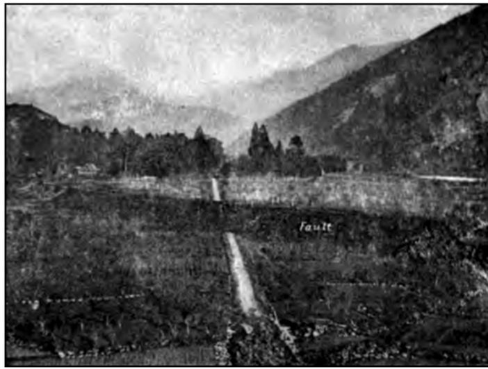
FIG. 47.—The Fault-scarp at Midori. ( Koto. )
