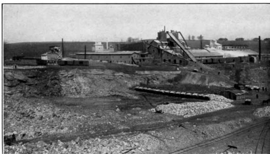
A Hydrated Lime Plant (Courtesy of the Palmer Lime and Cement Company, York, Pa.)
