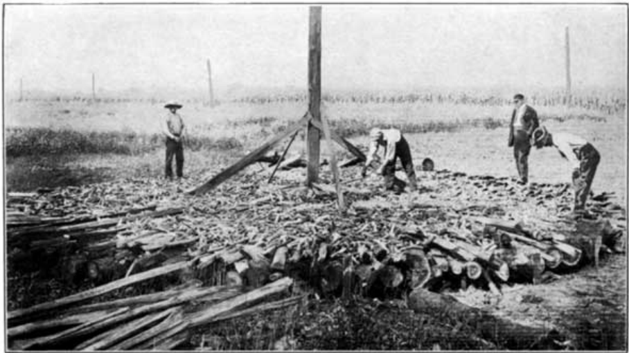
Laying Foundation for a Lime Stack at the Pennsylvania Experiment Station
