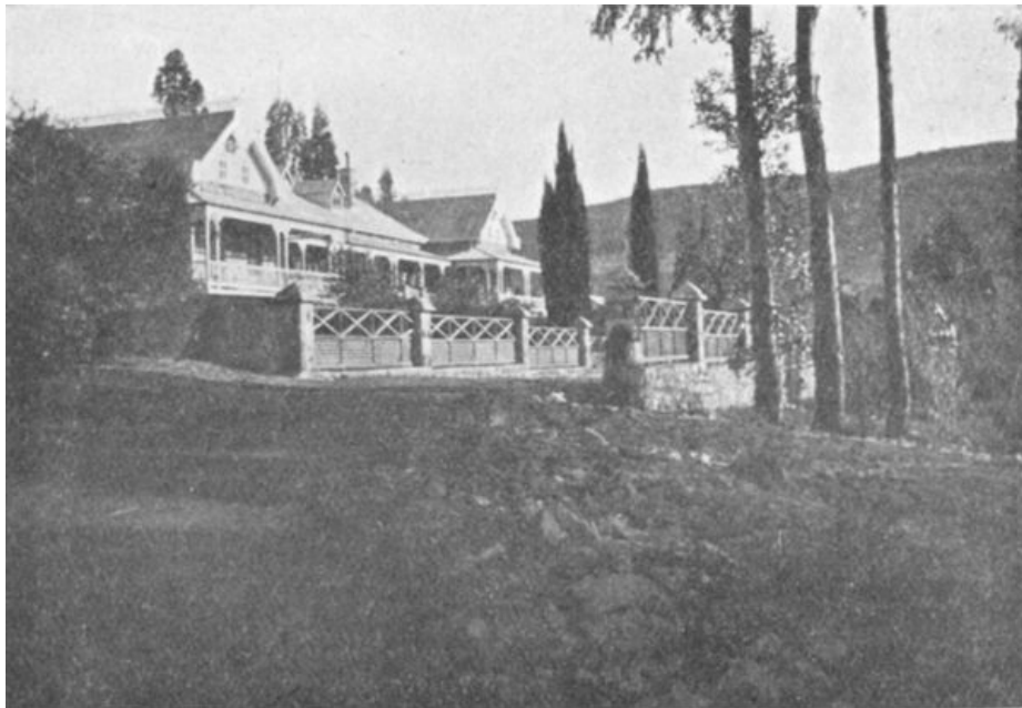
JOHAN MEYER'S HOUSE, FIVE MILES OUTSIDE JOHANNESBURG.
