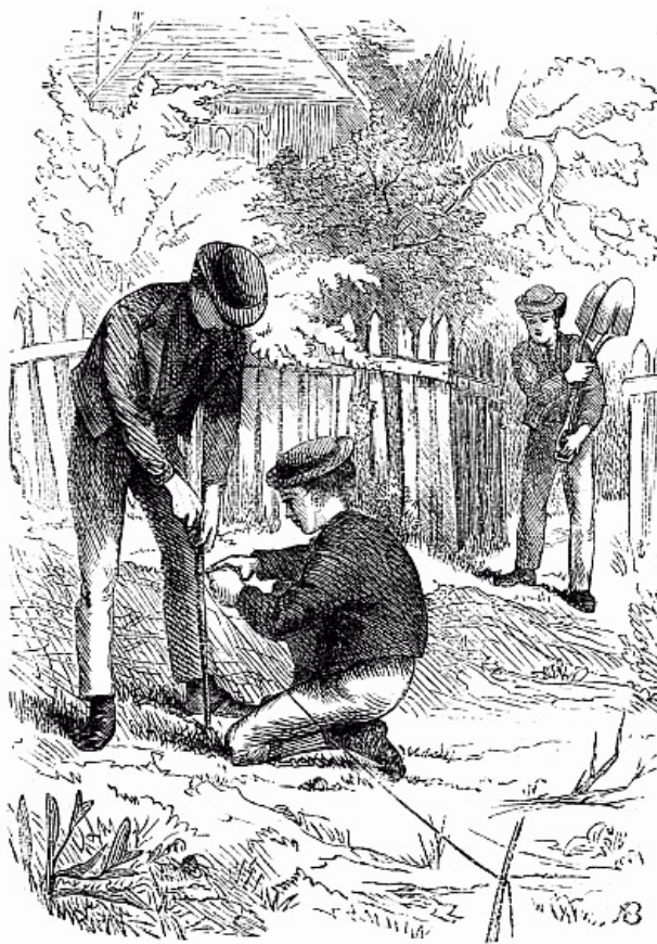
PLANNING OUT THE GROUND.
