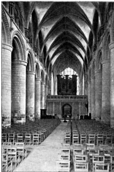
THE NAVE, LOOKING EAST.
