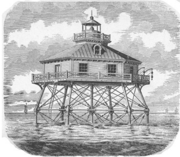
LIGHT-HOUSE AT “THE THIMBLE SHOAL,” HAMPTON ROADS, VA.
