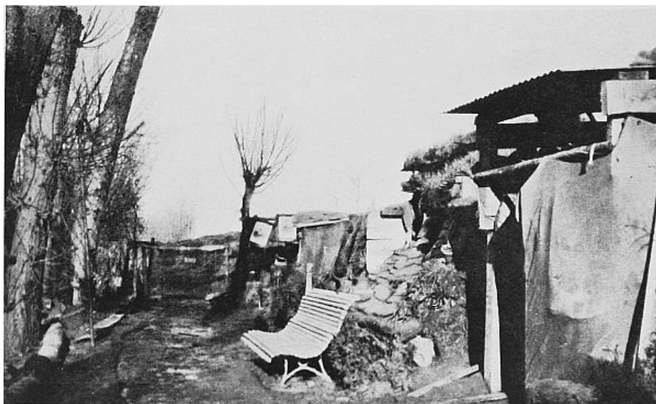
TRENCH BATTALION HEADQUARTERS. November, 1915—February, 1916.
