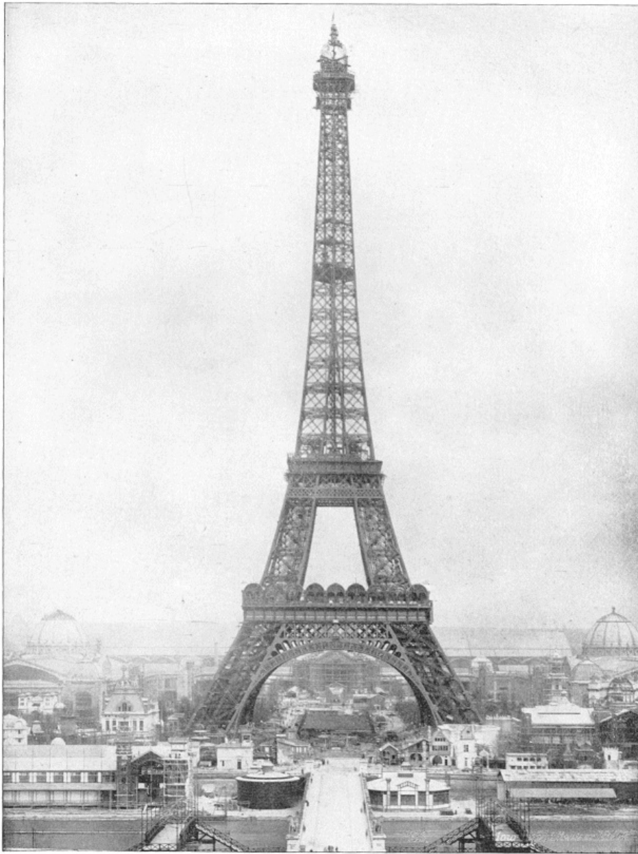
EIFFEL TOWER, PARIS, FRANCE.—This enormous monument surpasses anything of the kind hitherto erected. From all parts of the city its graceful head may be seen, completely dwarfing into insignificance every public building and spire that Paris contains. It has three platforms. The first, of vast extent and comfortably arranged for many hundred visitors at a time, contains cafés and restaurants. The second is 376 feet from the ground, and the third, 863 feet. The total height of the Tower is 985 feet, being the loftiest monument in the world.
