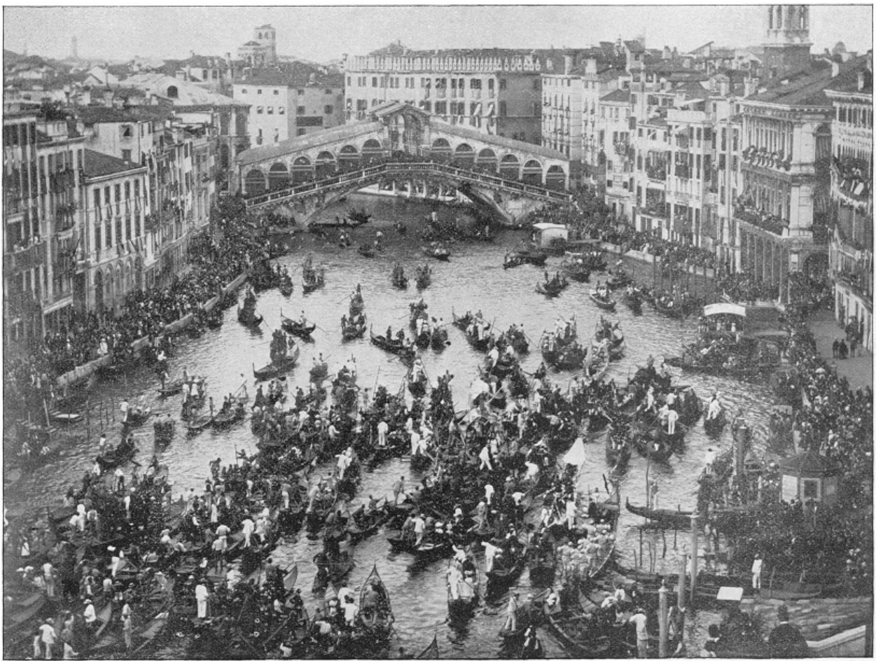
THE RIALTO, VENICE, ITALY.—This famous bridge, one hundred and fifty-eight feet long and forty-six feet wide, rests on twelve hundred posts. It was erected from 1588 to 1591. Its sides are lined with little shops, extending from a fish-market at one end, past jewelry-shops in the centre of the structure, down to a fruit-market at the other side. It always presents a busy appearance, and is considered a marvel of engineering skill, and one of the finest bridges in the world. The picture represents the annual parade on the Grand Canal, with the Rialto in the background, which is always the rallying centre on such occasions.
