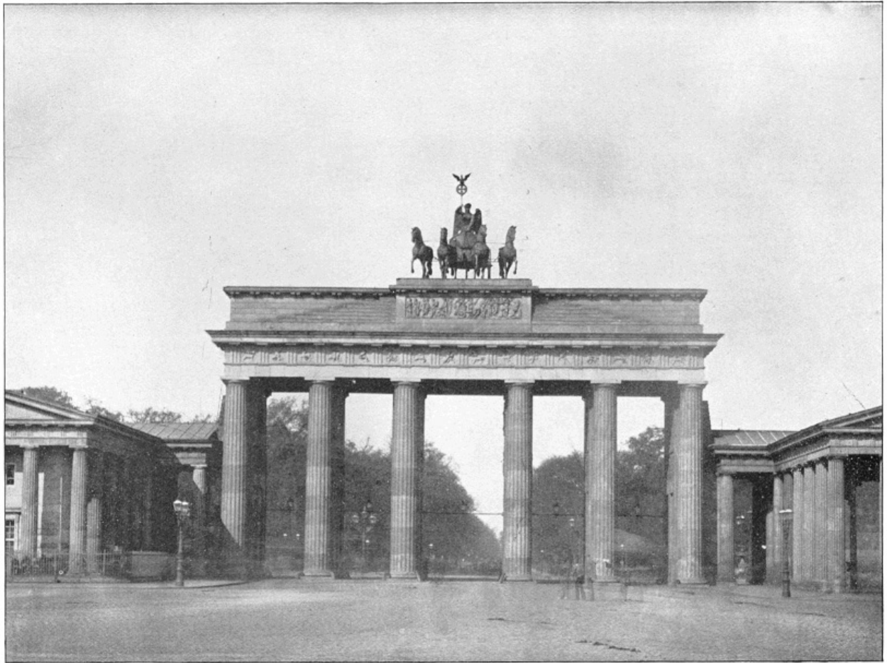
THE BRANDENBURG GATE, BERLIN, GERMANY.—The Brandenburg Gate, forming the entrance to Berlin, from the Thiergarten, was erected in 1793 in imitation of the Propylæa at Athens. It is 85 feet high and 205 feet wide, and has five different passages, separated by massive Doric columns. It is at the one end of "Unter den Linden," and its middle passage is reserved for royal carriages only. The material is sandstone, and it is surmounted by a Quadriga of Victory from copper, taken to Paris by Napoleon in 1807, but restored in 1814. On the side are two wings resembling Grecian Temples, one of which is a pneumatic post-office and the other a guard-house. Both combine in their construction, strength, elegance and beauty.
