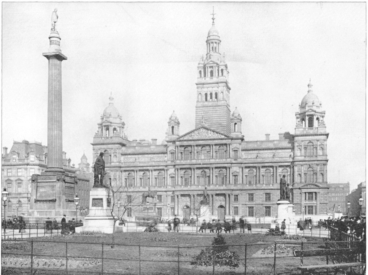
MUNICIPAL BUILDINGS, GLASGOW, SCOTLAND.—Glasgow is one of the best governed cities in Great
