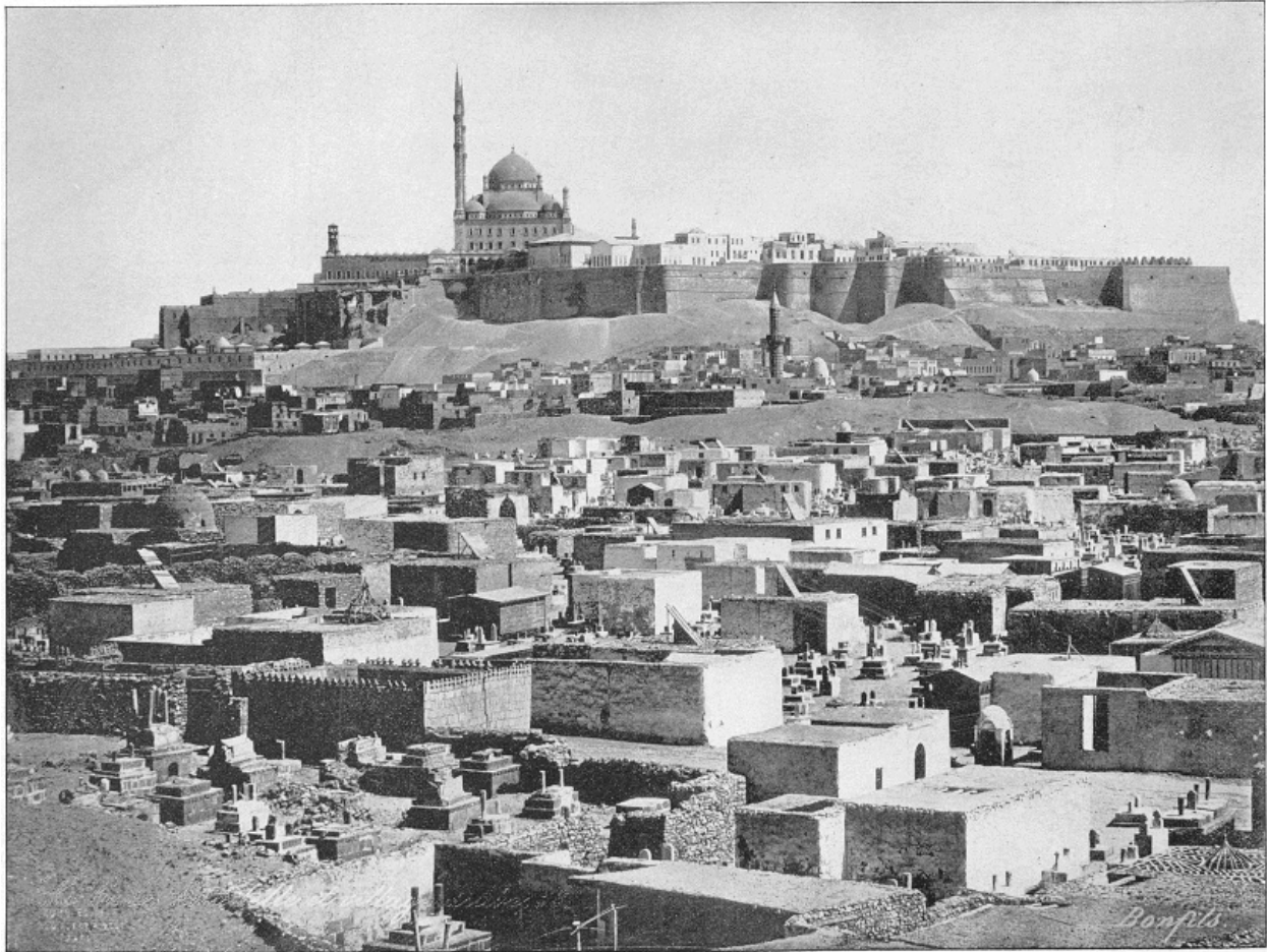
CITADEL, CAIRO, EGYPT.—This citadel affords a magnificent view of the city and surrounding country. It was erected in 1166, and built by stones taken from the small pyramids at Gizeh, the site having been selected, according to Arabian history, owing to the fact that meat could be kept here fresh twice as long as in any other part of Cairo. The fortress commands the city, yet its site is unfavorable, as a commanding height close by compelled its surrender during the wars of 1805.
