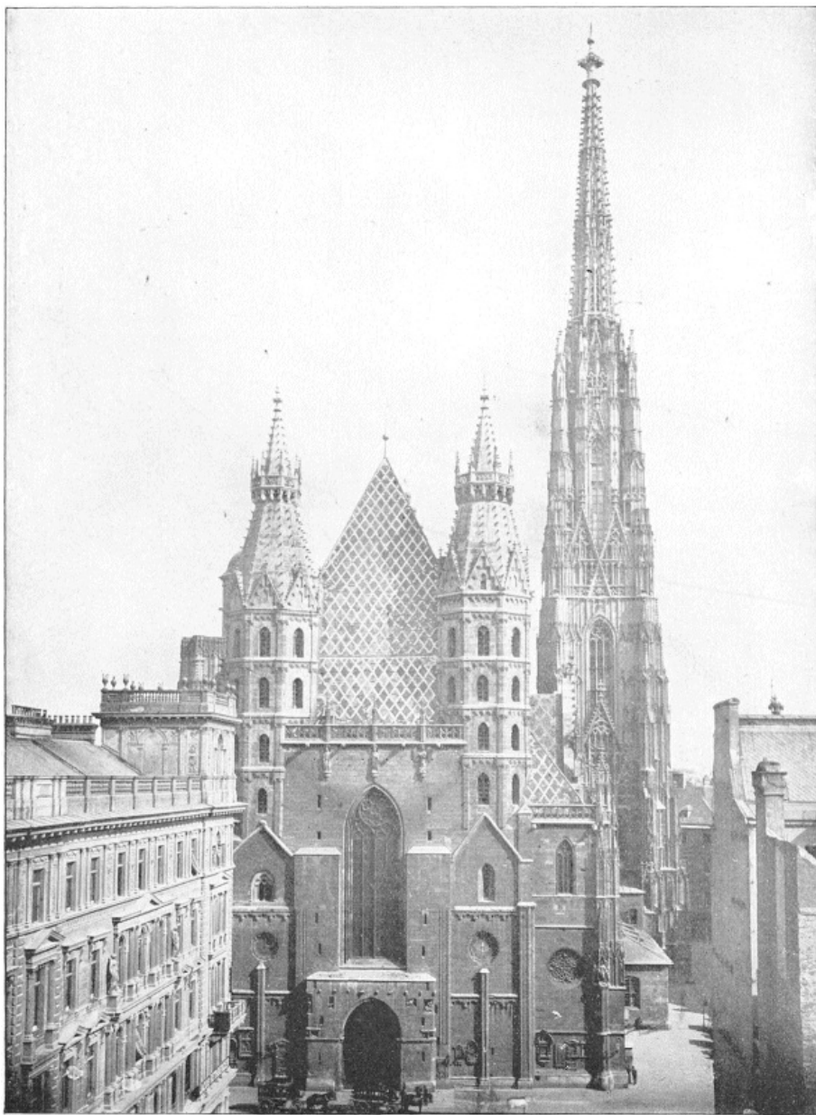
CHURCH OF ST. STEPHEN, VIENNA, AUSTRIA.—This is the most important edifice in the Austrian capital, dating back in its construction to the thirteenth century. It is constructed of solid limestone, and built in the form of a Latin cross. Below the church are extensive catacombs, consisting of three vaults, filled with bones and skulls. Centuries ago, the sovereigns of Austria were buried in these vaults. The Tower, built between 1860 and 1864, affords an extensive view, embracing the river Danube and the battle-fields of Loban, Wagram and Essling.
