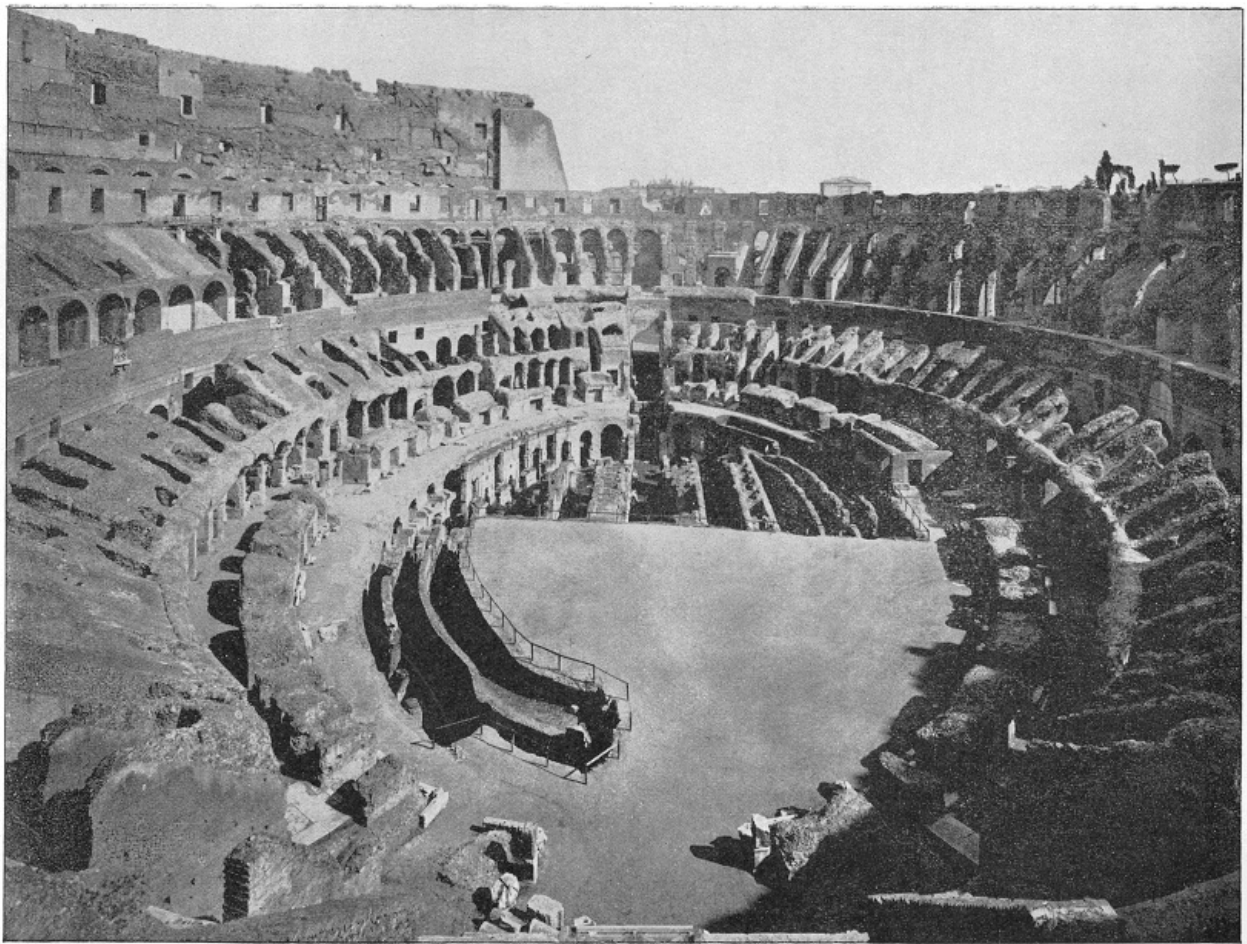
INTERIOR OF COLOSSEUM, ROME, ITALY.—The arches of the first tier are marked by Roman numbers, as they formed so many entrances, through which, by means of internal stairways, the upper balconies were reached. The Arena had two openings enclosed by railings of bronze, through which the gladiators and wild beasts entered. Above was the Podium, a place intended for the Emperors and their families, for the magistrates, the senators, the priests and the vestals. Thousands of Christians in this place suffered martyrdom, by becoming the prey of wild beasts. The picture presents the imposing spectacle of the interior of this monument at the present day.
