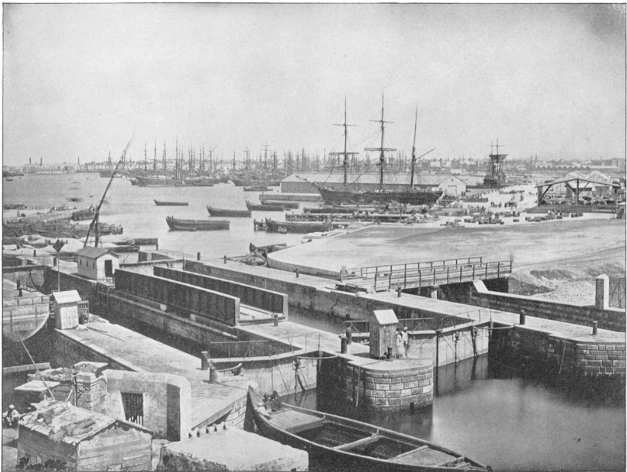
HARBOR, ALEXANDRIA, EGYPT.—The perfectly flat coast of Egypt, and even Alexandria itself, are not visible to the steam-boat passenger until very shortly before the vessel enters the harbor. The latter consists of an outer breakwater, forming an obtuse angle nearly two miles in length. A second pier, nearly a mile in length, protects an inner harbor covering nearly five hundred acres of water, twenty-seven feet deep. No fewer than thirty thousand artificial blocks, weighing twenty tons each, and two million tons of natural blocks of stone were used in the construction of these magnificent harbor works.
