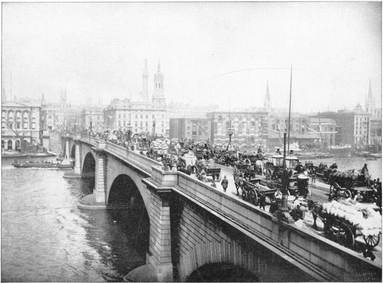
LONDON BRIDGE, LONDON, ENGLAND.—Centuries ago the Saxons and Romans erected various wooden bridges over the Thames, on the site of the present London Bridge; but they were all carried away by floods, or destroyed by fire. This bridge was begun in 1825 and completed in 1831 at a cost of $10,000,000. The bridge, 928 feet long and 54 feet wide, is borne by five granite arches, that in the centre having a span of 152 feet. The lamp-posts on the bridge are cast of the metal of French cannons captured in the Peninsular War. About 15,000 vehicles and 100,000 pedestrians cross the bridge daily.
