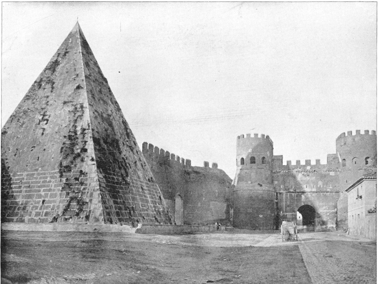
PYRAMID OF CESTIUS AND ST. PAUL GATE, ROME, ITALY.—The pyramid enclosed by Aurelian
