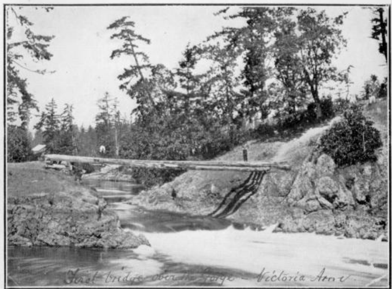
FIRST BRIDGE OVER THE GORGE, VICTORIA ARM.
