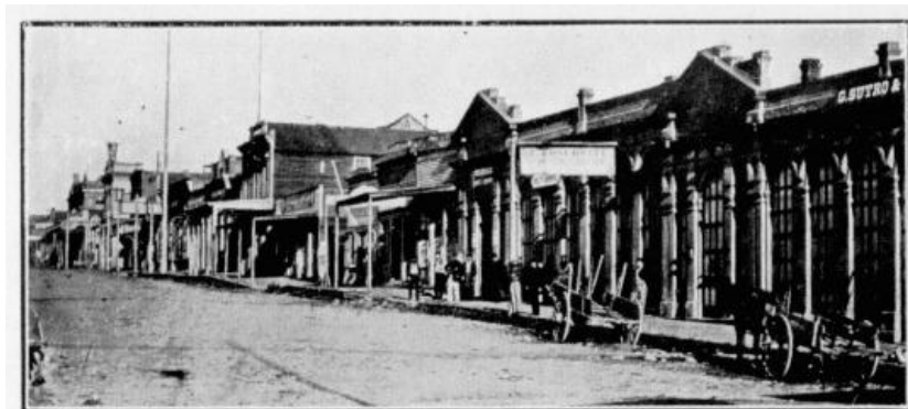
YATES STREET, LOOKING EAST.
