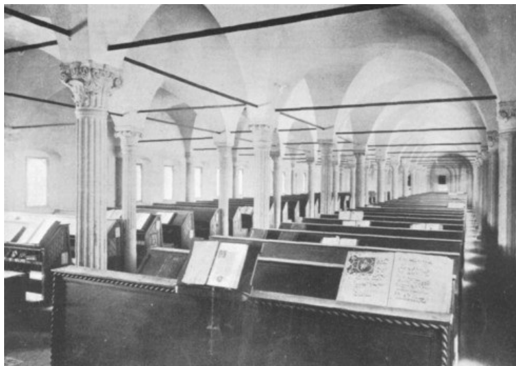
Fig. 92. General view of the Library at Cesena. From a photograph.
