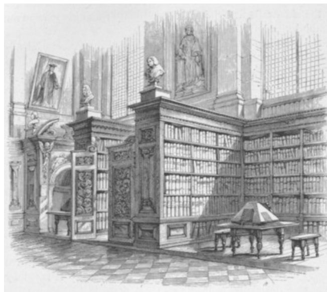
Fig. 128. Interior of the north-east corner of the Library of Trinity College, Cambridge, shewing the bookcases, table, desk and chairs, as designed by Sir C. Wren.
