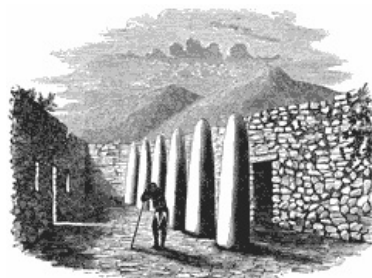
Fig. 31.—Great Hall at Mitla.
