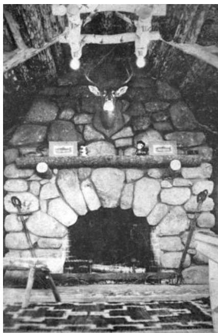
A fireplace and chimney breast of field stone, chosen with care and laid with more than average skill
