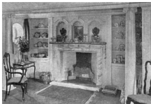
One of the best forms of the basket grate in brass. The splayed sides send out more heat
