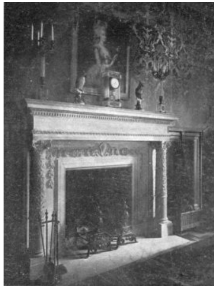
Caen stone or its clever representation in cement serves well for the more formal type of mantel and facing
