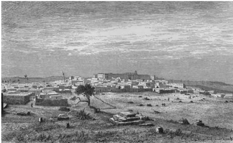
EL HARISH (VIEW ON THE NORTHERN SIDE).
