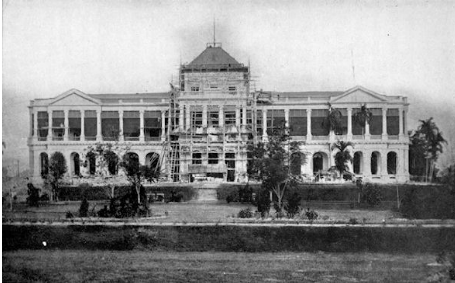
GOVERNMENT HOUSE, SINGAPORE, APPROACHING COMPLETION.
