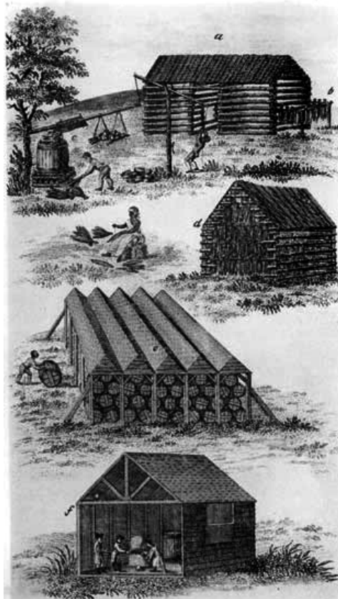
PLANTATION TOBACCO HOUSES AND PUBLIC WAREHOUSES a, The common tobacco house. b, Tobacco hanging on a scaffold. c, The operation of prizing. d, Inside of a tobacco house, showing the tobacco hanging to cure. e, An outside view of a public warehouse. f, showing the process of inspection.
