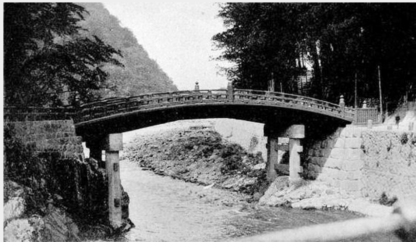
PLATE IV Sacred Red Bridge at Nikko. Legend Says It Was Built for the Saint Shodo Shonin. No One Crossed It Except the Shoguns and in Modern Times the Mikado. General Grant Was Given a Permit to Cross This Bridge, but Sensibly Refused to Use It
