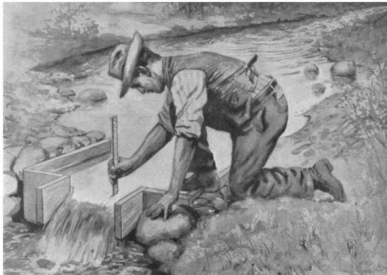
Measuring a small stream with a weir
