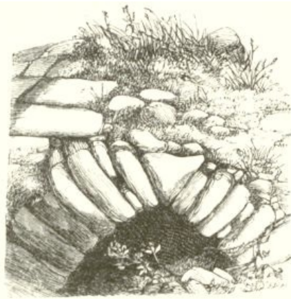
Fig. 9. Exposed section of the arch of the vault.
