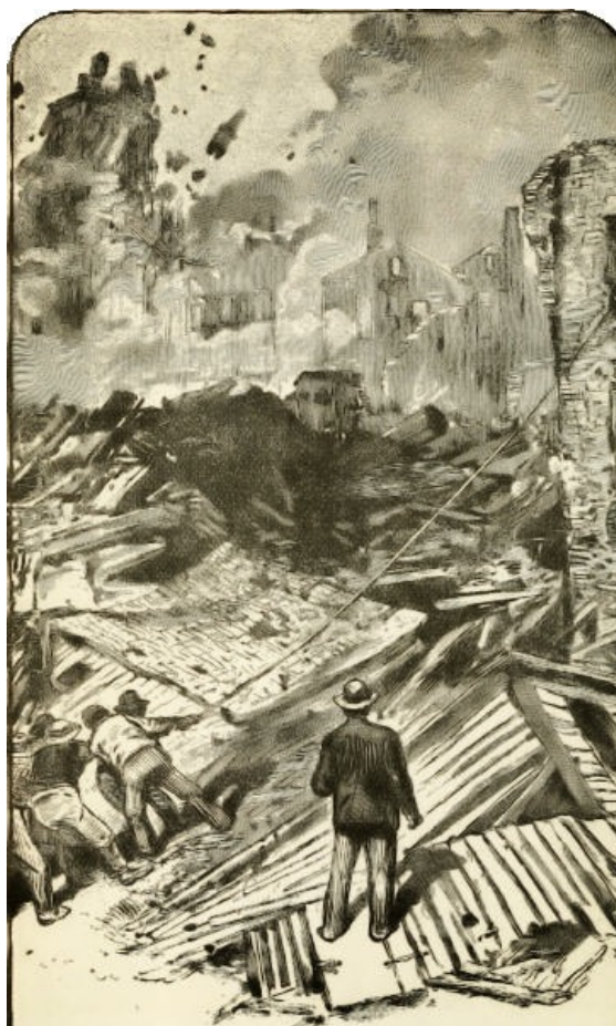
TEARING DOWN HOUSES IN JOHNSTOWN.
