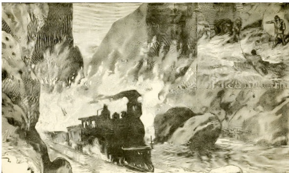
A GRAVEL-TRAIN RUNS AWAY FROM THE ADVANCING FLOOD.
