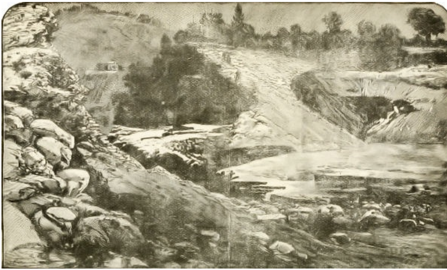
IMMENSE GAP IN THE BROKEN DAM, AS SEEN FROM THE INSIDE.
