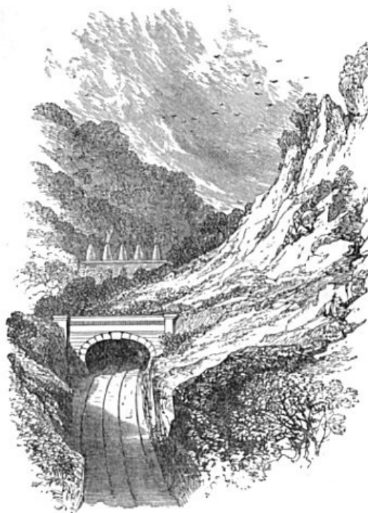
Land-slip on North Midland Line, near Ambergate.
