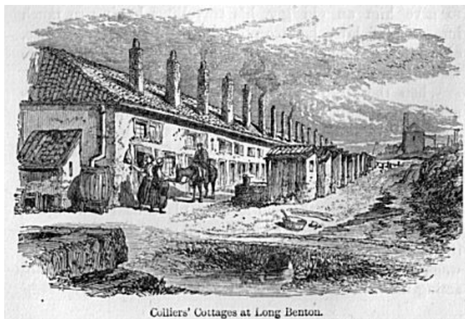
Colliers' Cottages at Long Benton.
