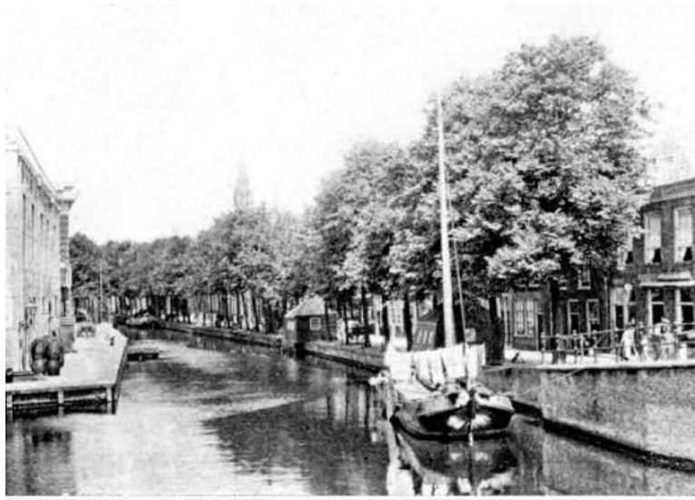
Near the Arsenal, Delft
