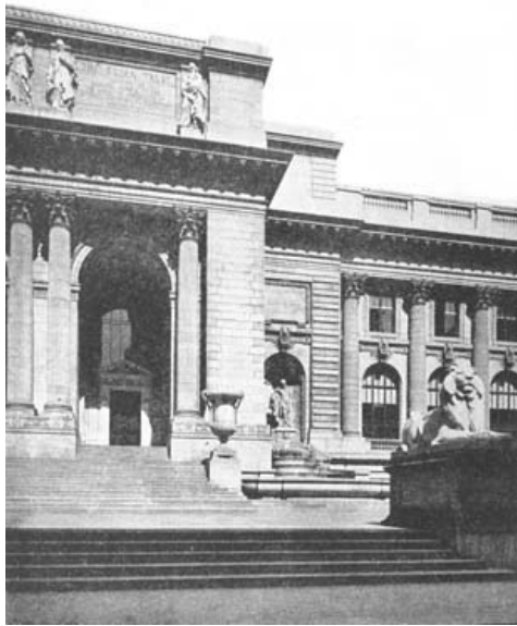
PART OF MAIN FAÇADE
