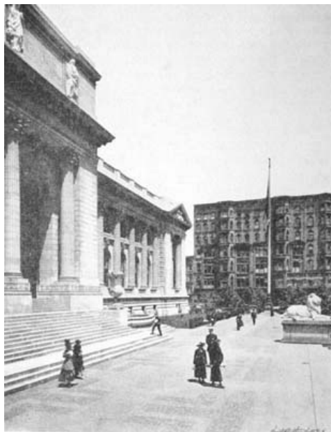
TERRACE LOOKING NORTH
