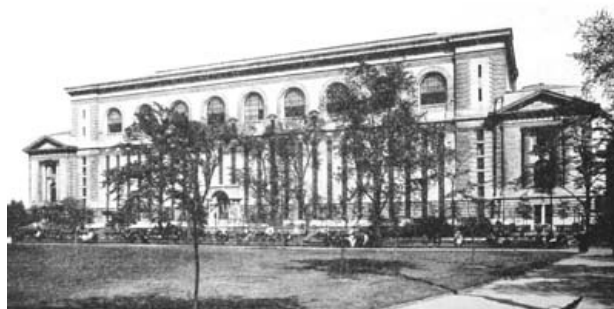
REAR OF LIBRARY FROM BRYANT PARK
