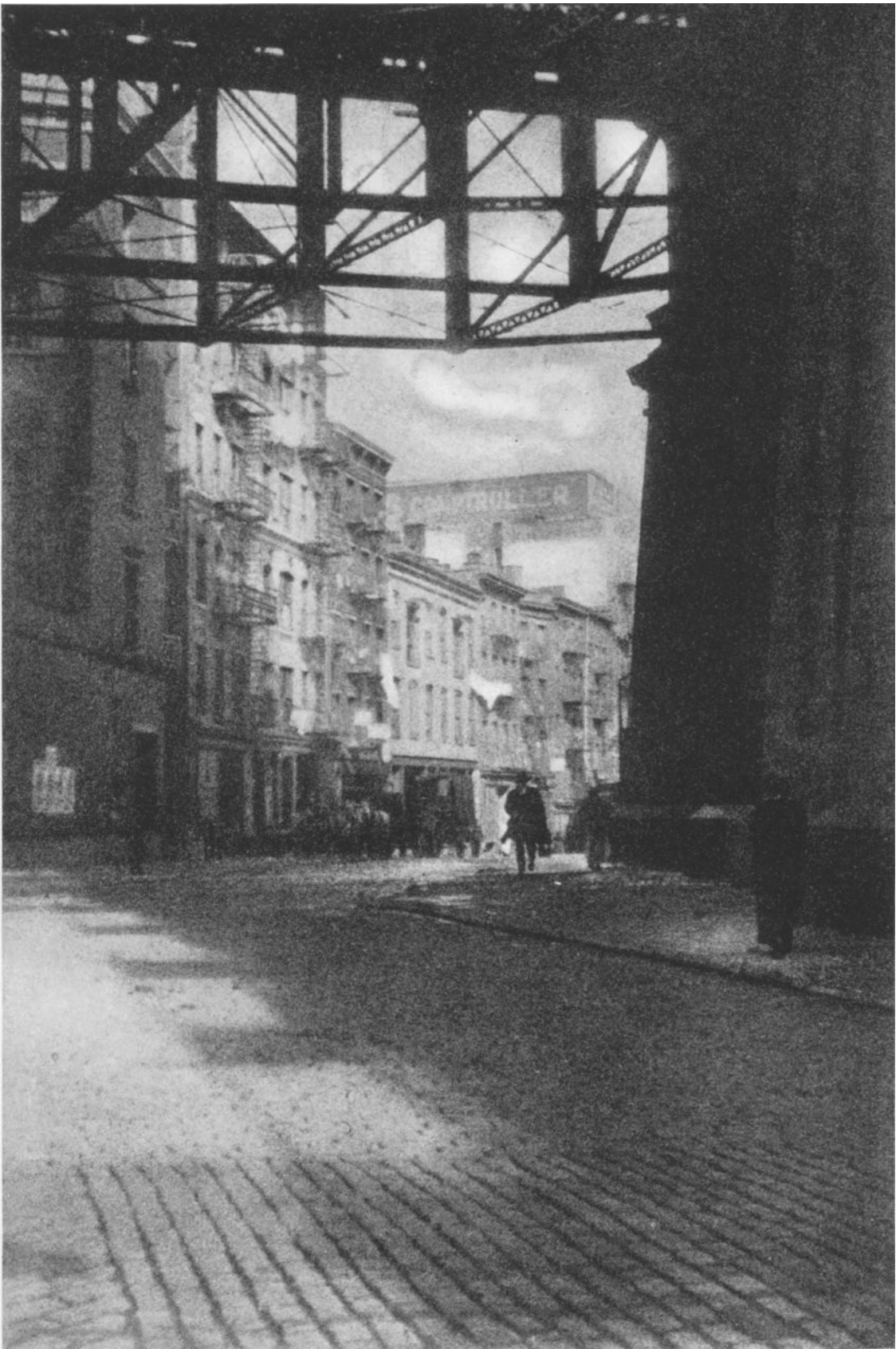
UNDER BROOKLYN BRIDGE By A. E. SCHAAF, Cleveland, Ohio
