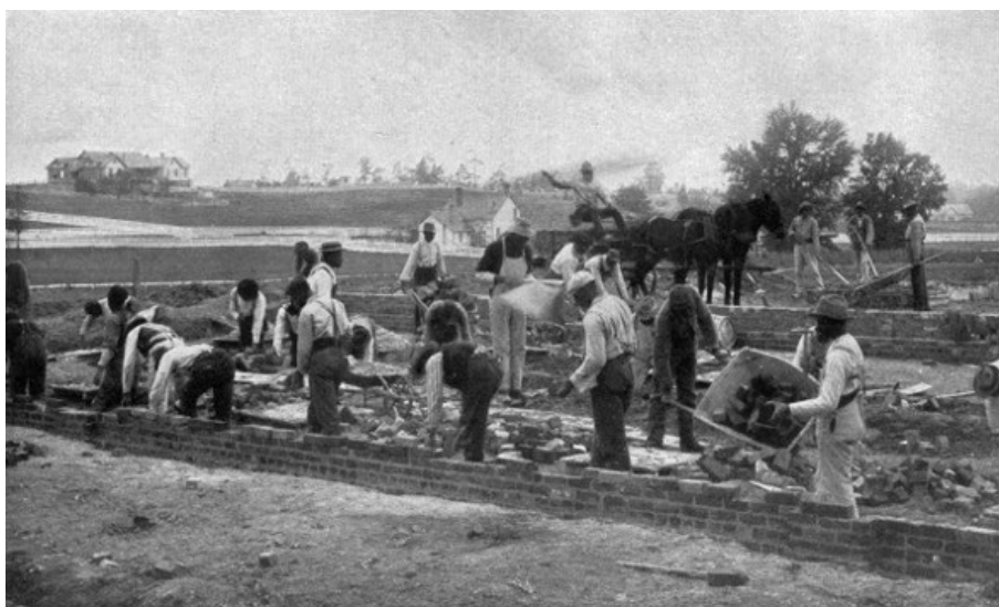
STARTING A NEW BUILDING. Student masons laying the foundation in brick.
