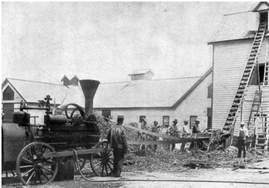
A SILO ON THE FARM. Students filling it with fodder corn, steam-power being used.
