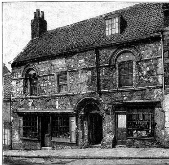
Norman House at Lincoln, called the Jews' House. Built about 1140. The square windows are of later date.
