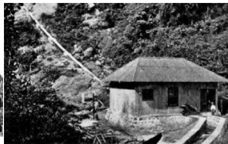
Hydro-electric power plant on Finca Ona.
