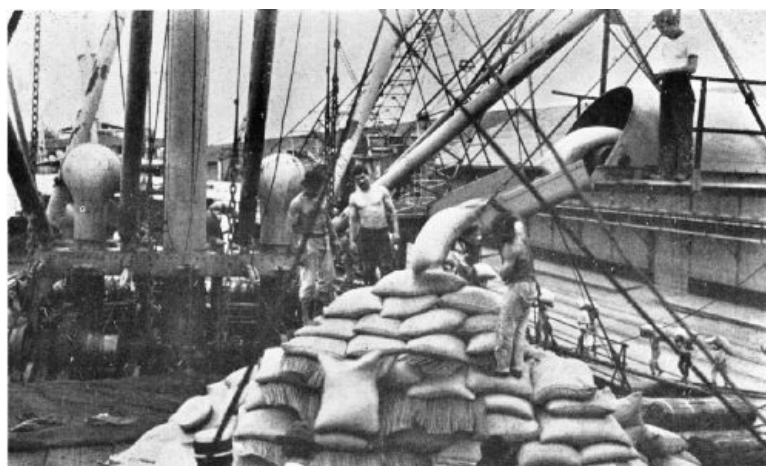
HERE THE AUTOMATIC BELT POURS INTO THE HOLD A CONTINUOUS STREAM OF BAGS OF COFFEE OLD AND NEW METHODS OF LOADING COFFEE AT SANTOS
