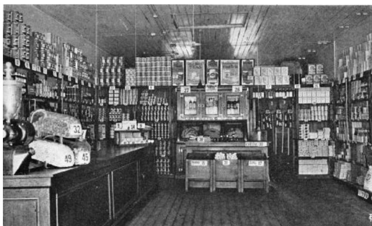
TYPICAL CHAIN-STORE INTERIOR EQUIPMENT
