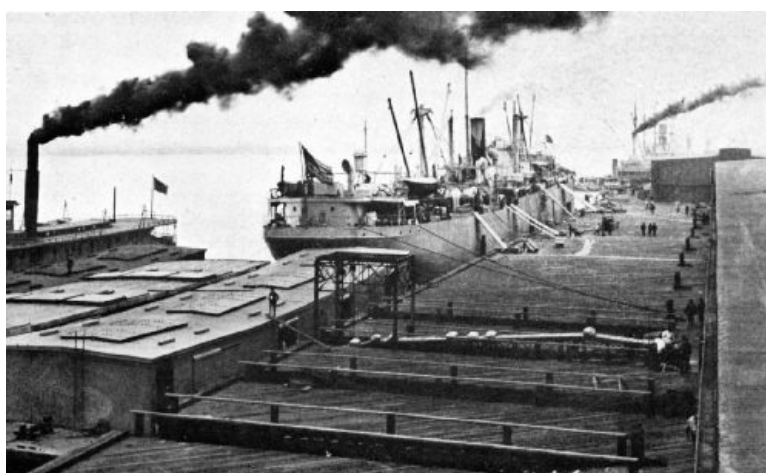
IN FOREGROUND—LOADING COFFEE BY MEANS OF AN AUTOMATIC TRAVELING-BELT CONVEYOR, ON GOVERNMENT BARGES FOR ST. LOUIS COFFEE-HANDLING SCENES ON THE WHARVES AT NEW ORLEANS
