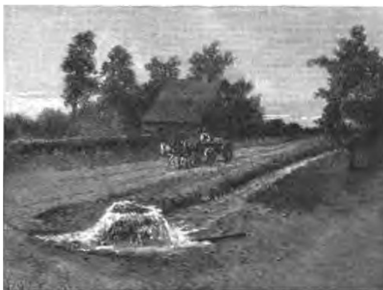
IRRIGATION BY PIPE SYSTEM.
