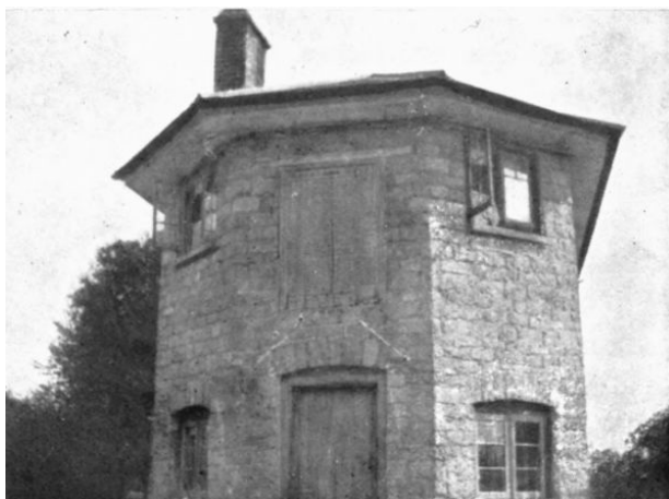
BAGSTONE TURNPIKE GATE HOUSE. GATE ABOLISHED ABOUT 1870.
