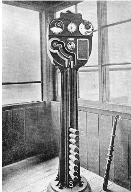
FIG. 101.—An electric train staff holder: s s, staffs in the slot of the instrument. Leaning against the side of the cabin is a staff showing the key \kappa at the end for unlocking a siding points between two stations. The engine driver cannot remove the staff until the points have been locked again.
