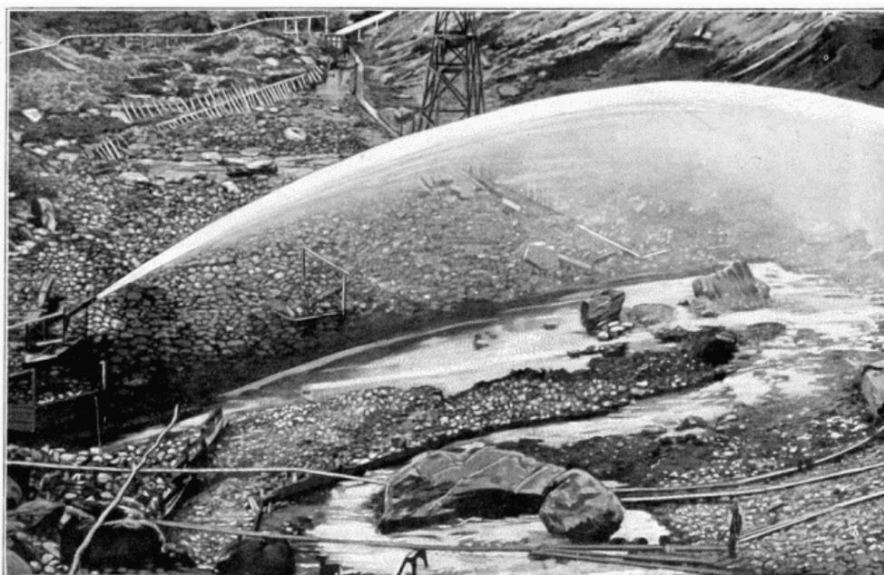
EXPLOITATION D'UN PLACER PAR LA MÉTHODE HYDRAULIQUE.—PHOTOGRAPHIE DE LA ROCHE À SEATTLE.
