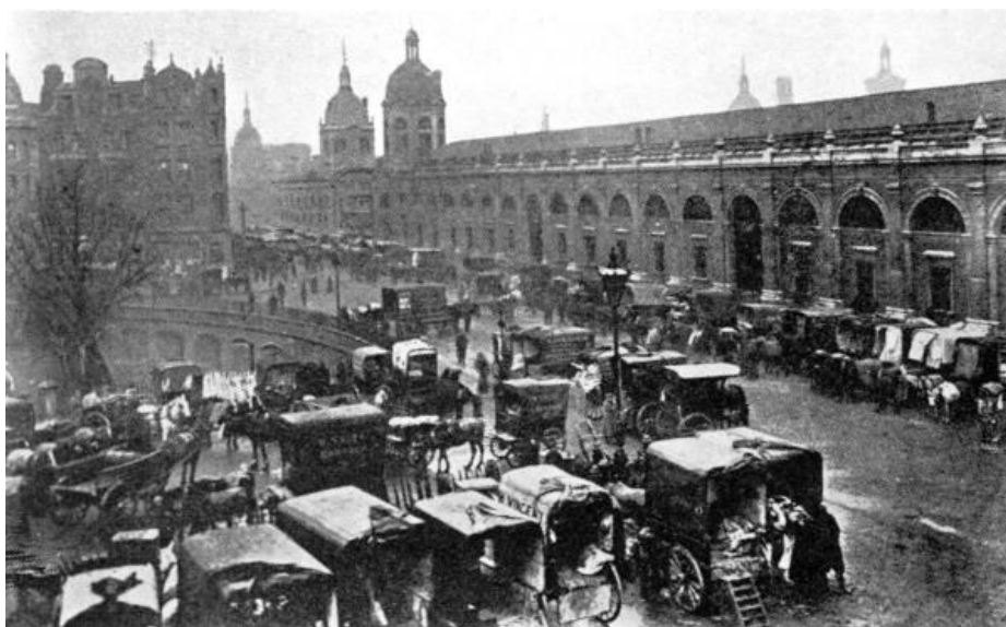
DELIVERING MEAT AT SMITHFIELD TODAY There is an inclined road by the tree in the center of the picture, leading to the special railroad freight depot. Cars are also run directly under the market and their cargoes are delivered by hydraulic lifts to the stands above.
