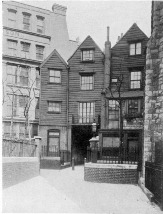
OLD WOODEN HOUSES AT CRIPPLEGATE (RECENTLY DEMOLISHED).
