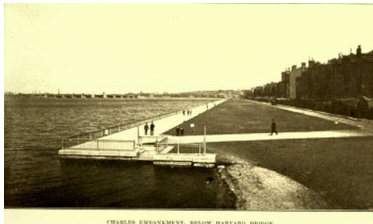
CHARLES EMBANKMENT, BELOW HARVARD BRIDGE
