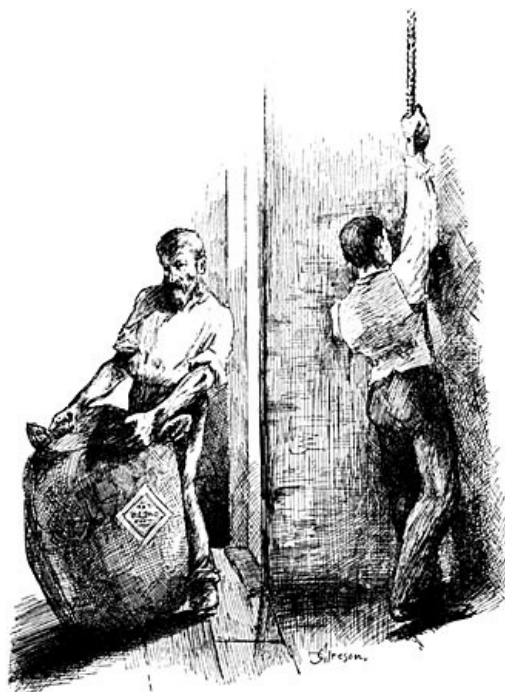
HERBERT RANDOLPH WORKING ON THE HOIST.
