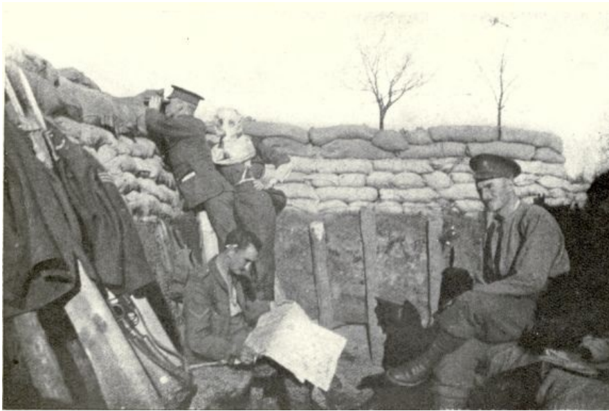
OUR TRENCHES AT PLUGSTREET.
