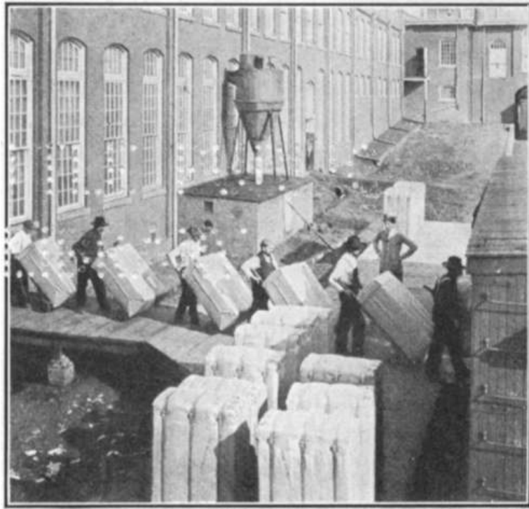
Baled cloth being put aboard waiting freight cars
