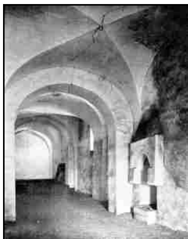
S. SAVIOUR PANTOKRATOR. GALLERY OF THE NORTH CHURCH, LOOKING SOUTH.
