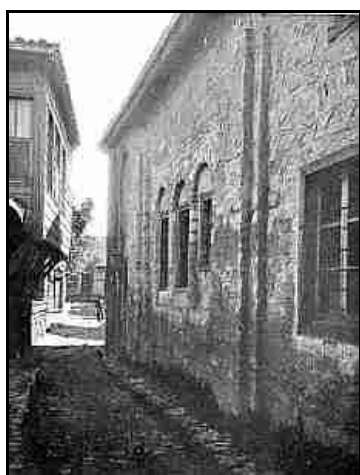
S. THEKLA. NORTH SIDE, FROM THE NORTH-WEST.
