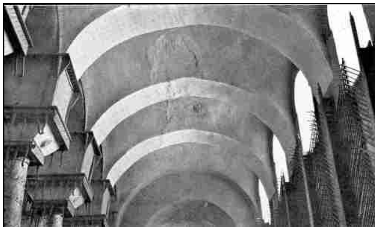
S. IRENE. VAULTING OVER THE SOUTH AISLE.
