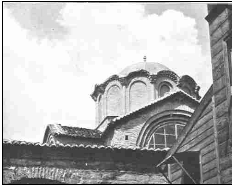
S. THEODORE. THE CENTRAL DOME, FROM THE SOUTH
