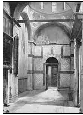
S. SAVIOUR IN THE CHORA. THE INNER NARTHEX, LOOKING SOUTH.
