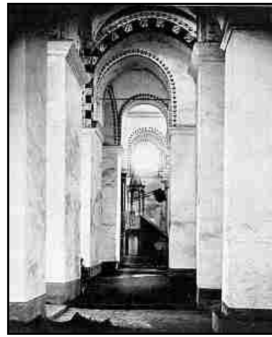
S. SAVIOUR PANTOKRATOR. THE INTERIOR, LOOKING FROM THE SOUTH CHURCH THROUGH INTO THE NORTH CHURCH.
