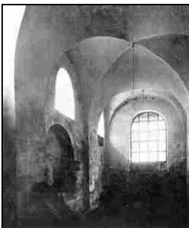
S. SAVIOUR PANTOKRATOR. NARTHEX OF THE NORTH CHURCH, LOOKING NORTH.
