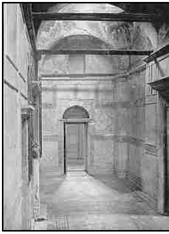
S. SAVIOUR IN THE CHORA. THE INNER NARTHEX, LOOKING SOUTH.
