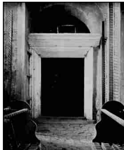
S. IRENE. DOOR AT THE EAST END OF THE NORTH AISLE.
