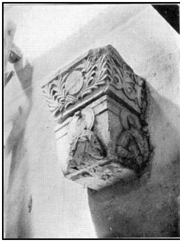
S. SAVIOUR IN THE CHORA. BRACKET IN THE INNER NARTHEX INTERIOR, LOOKING EAST.
