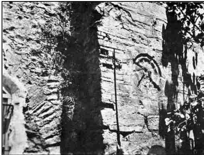
S. SAVIOUR PANTEOPTES. EXTERIOR DECORATION IN BRICK, ON SOUTH SIDE
