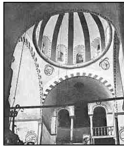
S. SAVIOUR PANTEPOPTES. THE DOME, LOOKING WEST.
